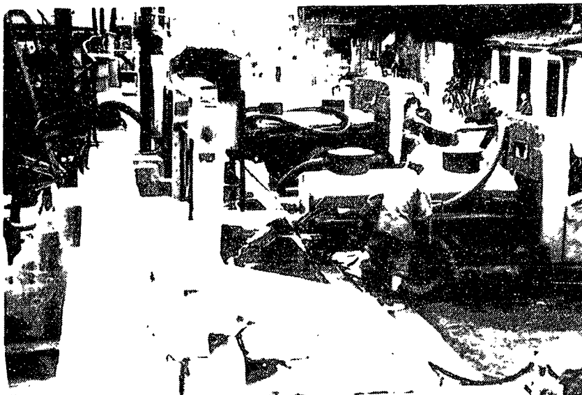
Figure 1.3 Night soil in Shanghai is pumped from riverside storage tanks into barges for transport to rural areas for reuse.
