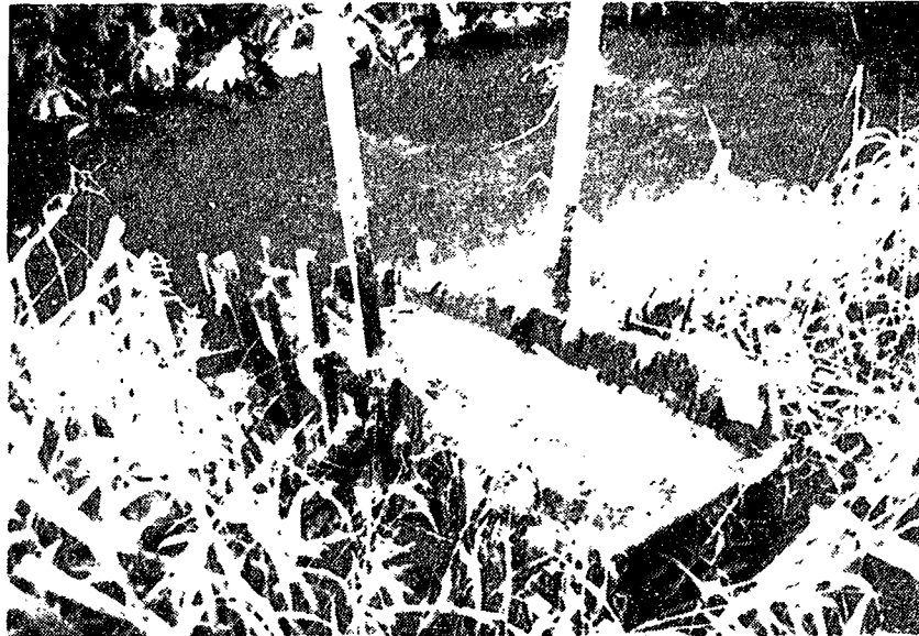
Figure 2.5 In Malaysia, night soil is loaded into a pond using a wooden chute
