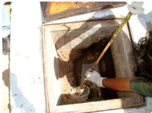
Removal of obstacle from the sewer pipeline
