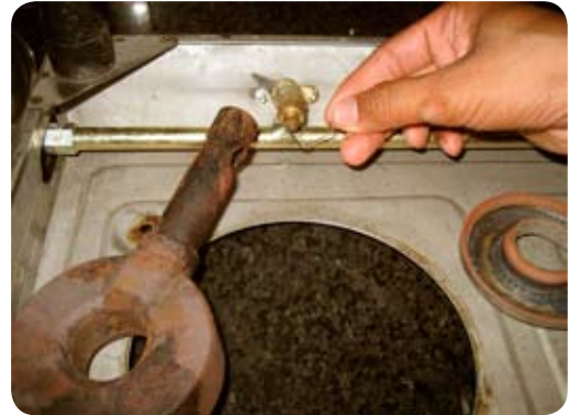
Cleaning of Jet holes
