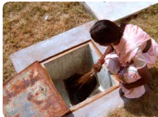
Cleaning of inspection chambers
