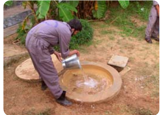
Filling water to required depth
