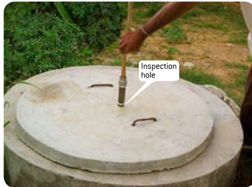
Checking the level of water seal
