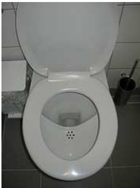
Figure 3 Roediger Vacuum urine-diversion flush toilet and Keramag urinal (flickr, 2011)
