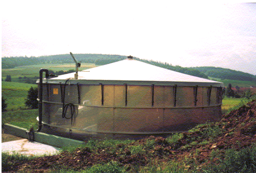
Figure 9 Stainless steel tank (devosagri, 2011)
