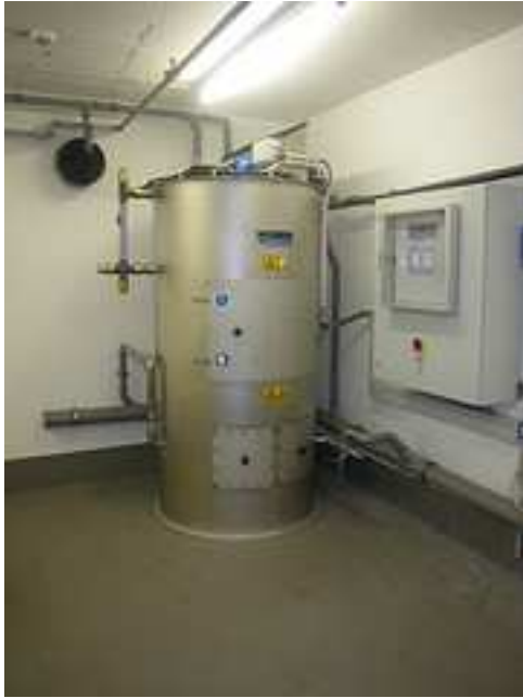
Figure 4 Magnesium–Ammonium–Phosphate precipitation reactor (flickr, 2011)
