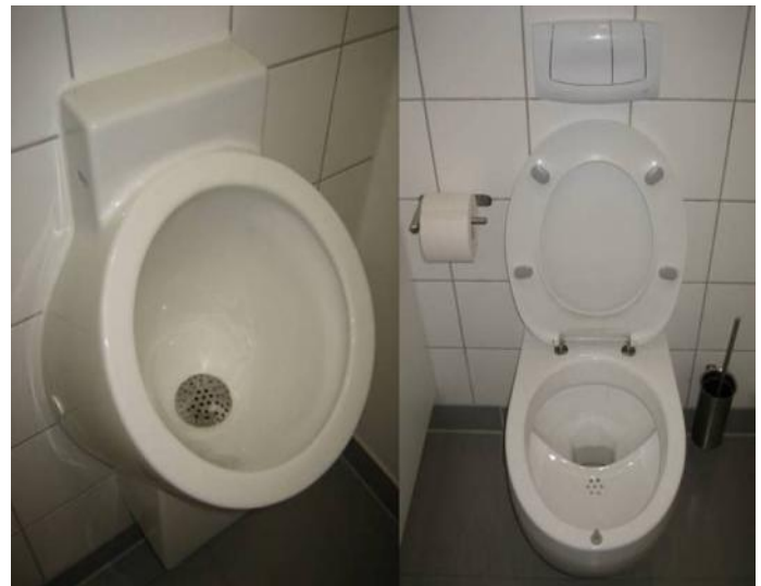
Fig. 4: Left: waterless urinal (Keramag). Right: urine-diversion flush toilet (Roediger) at GIZ main building; note the two buttons for flushing: the small one is for the urine flush, the larger one for the faeces flush (source: L. Ulrich, January 2009).
