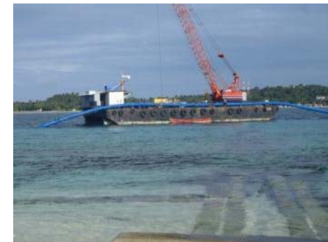
Construction of New Submarine Pipeline
