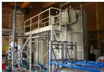
Waste Water Treatment facility
