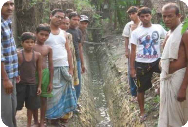
Cleaning up of Clogged Drains
