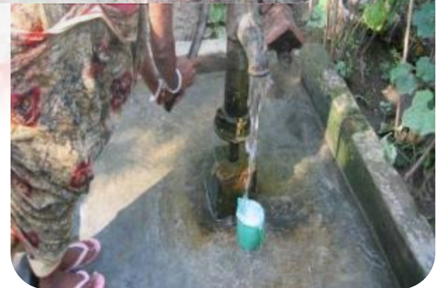
Hand pumps were established near to the toilet
