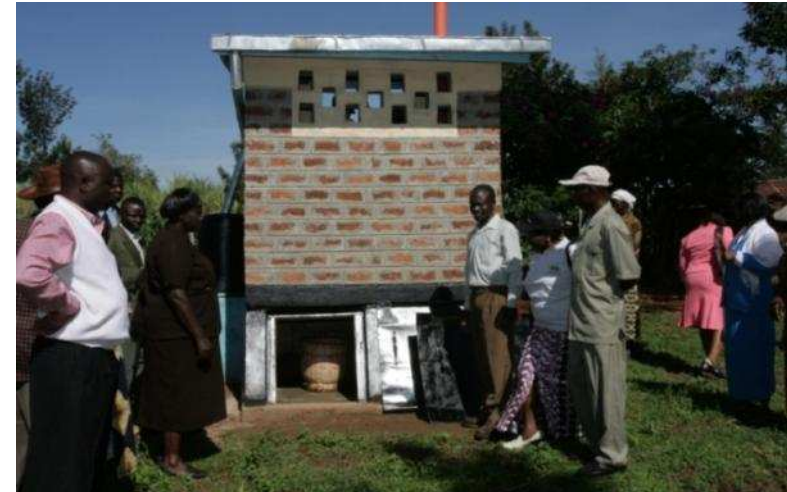
Urine Diverting De-hydrating Toilets - UDDTs
