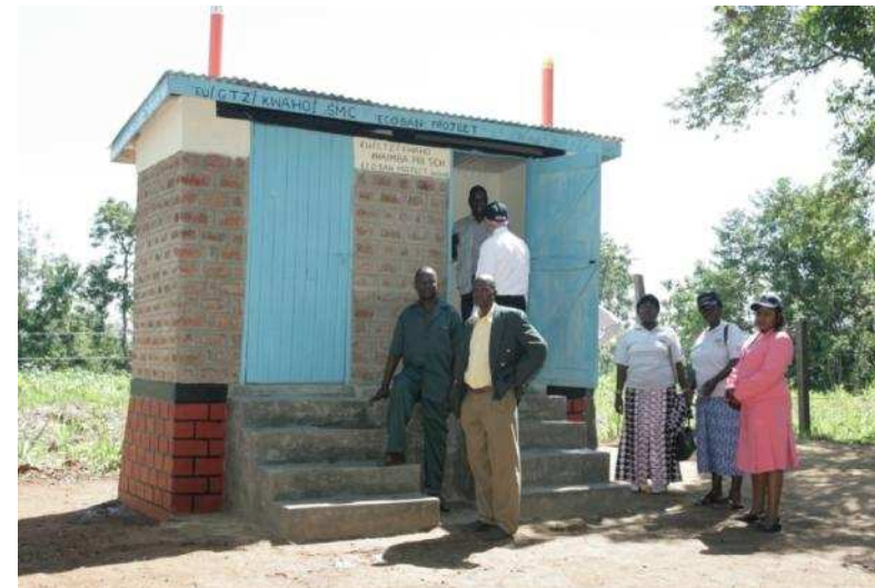
Urine Diverting De-hydrating Toilets - UDDTs
