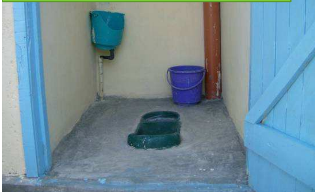
Inside of a UDDT piloted by ROSA at the household level
