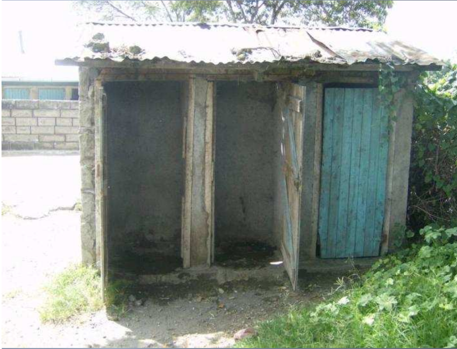
An existing (pit) sanitation facility
