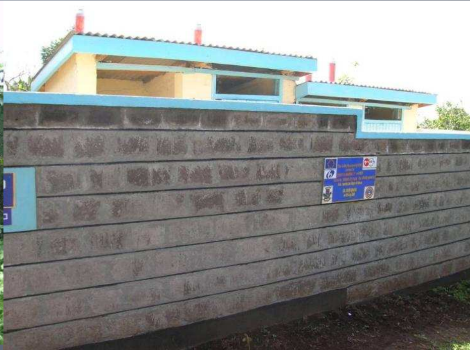
A ROSA UDDT constructed ecosan facility
