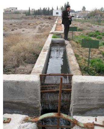
Simple screens for wastewater screening
