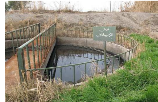
Circular primary settling tank
