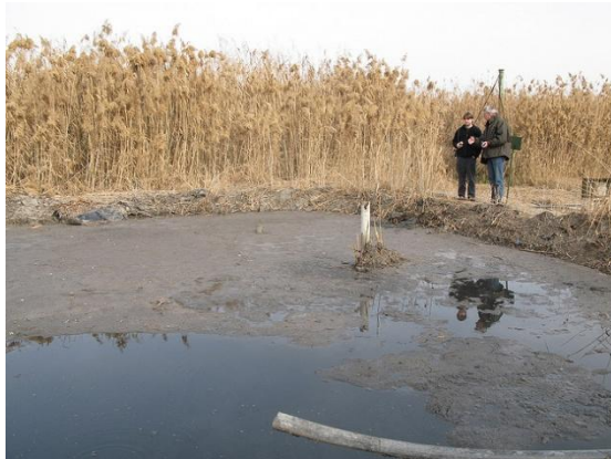
Primary sludge drying bed in front of reed bed. At the front you can see the sludge pipe from the primary settling tank.
