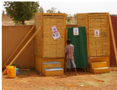
The door is a bit heavy, so sometimes the walls need extra support.
