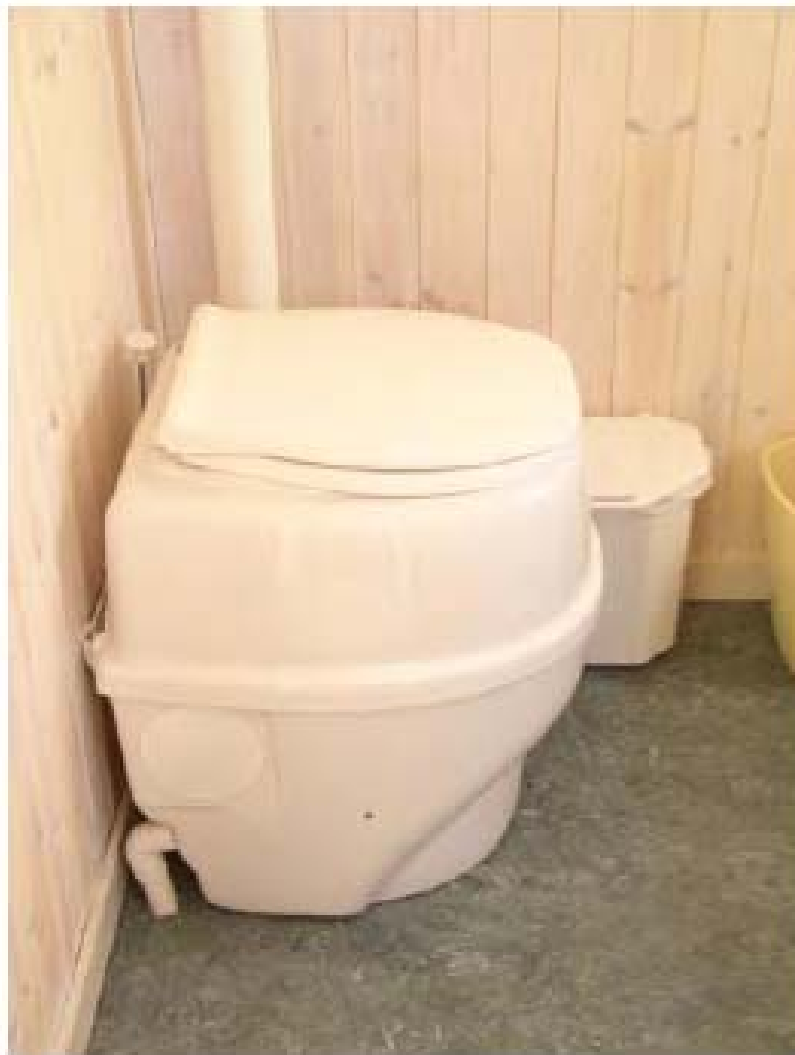
Figure 2. Urine diversion in the on-site low population density context. a) South Africa, photo: Aussie Austin b). Sweden, Separett is a dry urine diverting toilet for indoor use. Photo: Mats Johansson.
