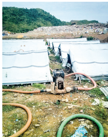
ABOVE: One of two emergency waste management sites in Yolanda-affected areas was located in the Municipality of Palo, Leyte. Mixing cells were constructed using coconut lumber (FAR LEFT), lined with plastic, filled with fecal sludge and mixed with lime (LEFT CENTER); the waste was then pumped (RIGHT CENTER) to one of many drying beds (FAR RIGHT) to conclude treatment.
