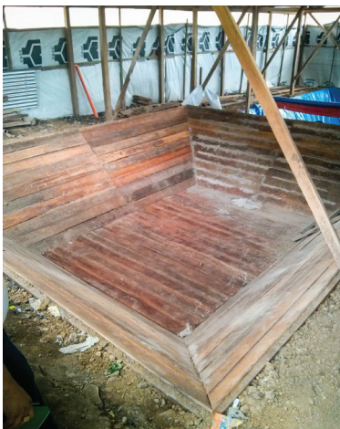
ABOVE: One of two emergency waste management sites in Yolanda-affected areas was located in the Municipality of Palo, Leyte. Mixing cells were constructed using coconut lumber (FAR LEFT), lined with plastic, filled with fecal sludge and mixed with lime (LEFT CENTER); the waste was then pumped (RIGHT CENTER) to one of many drying beds (FAR RIGHT) to conclude treatment.
