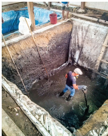
ABOVE: One of two emergency waste management sites in Yolanda-affected areas was located in the Municipality of Palo, Leyte. Mixing cells were constructed using coconut lumber (FAR LEFT), lined with plastic, filled with fecal sludge and mixed with lime (LEFT CENTER); the waste was then pumped (RIGHT CENTER) to one of many drying beds (FAR RIGHT) to conclude treatment.
