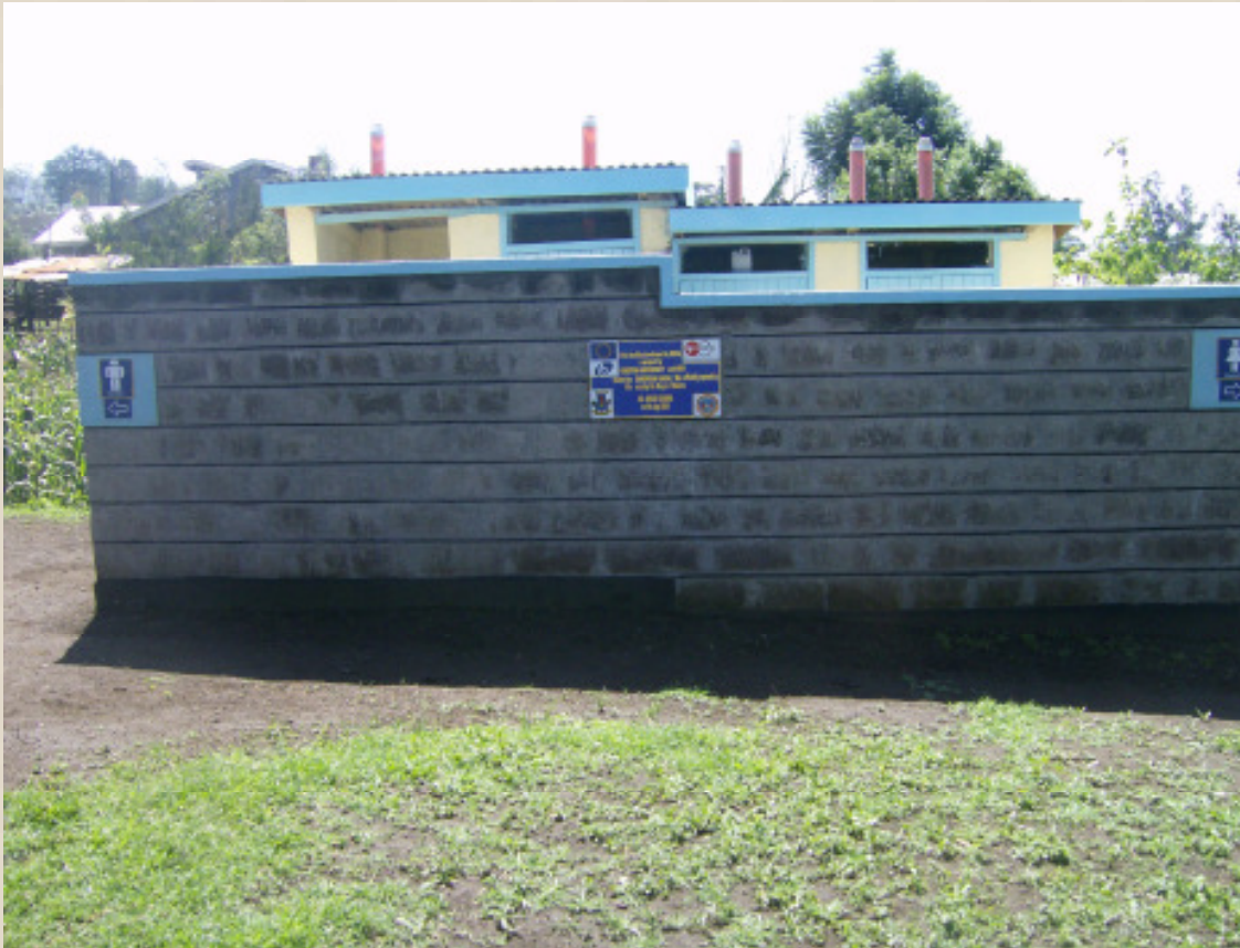
Pilot Unit at a Church/Nursery school
