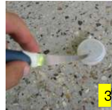
3 Cut hole in plug, smaller than hose
