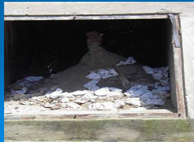
The inside of a toilet chamber. Kabale
