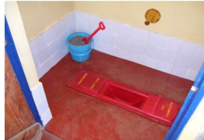
Squatting pan inside the toilets
