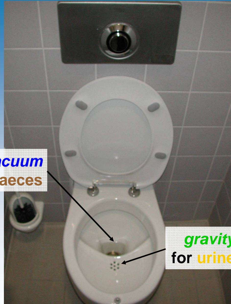
Roediger Vacuum Separation Toilet at WWTP Stahnsdorf
