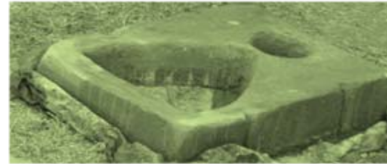
EcoSan squatting pan – Promoted by Water and Environmental Project Management organization (WEPMO). Photo by EEPCO 2007.
