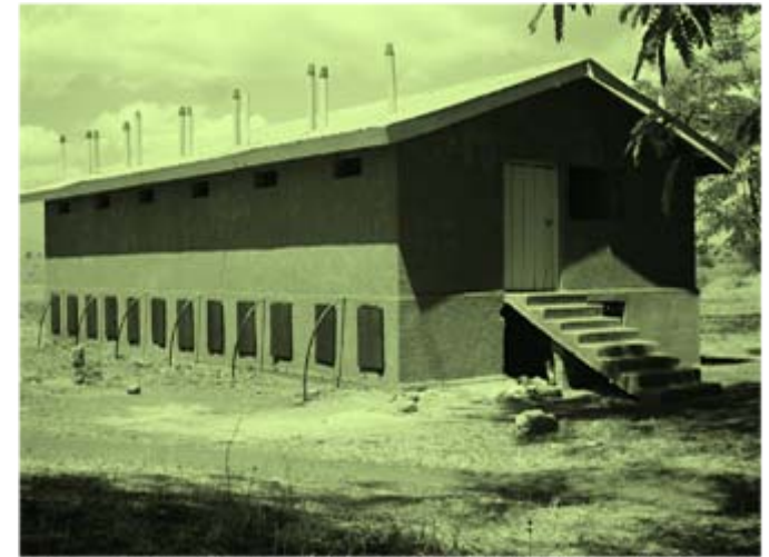
EcoSan School Toilet at Bomango'mbe – Hai District Kilimanjaro (photo by EEPCO 20002)
