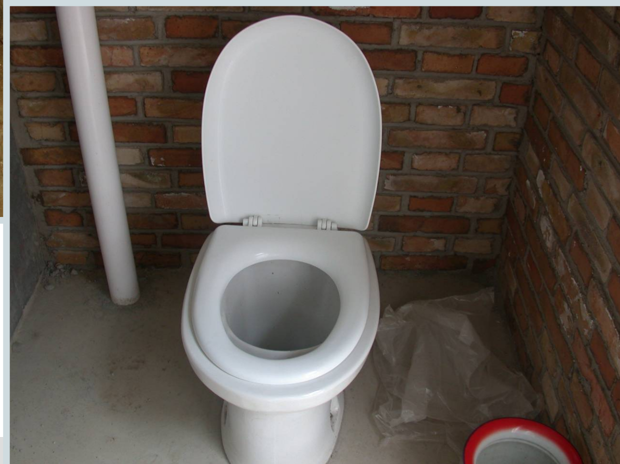
Before and after ecosan toilet renovation.
