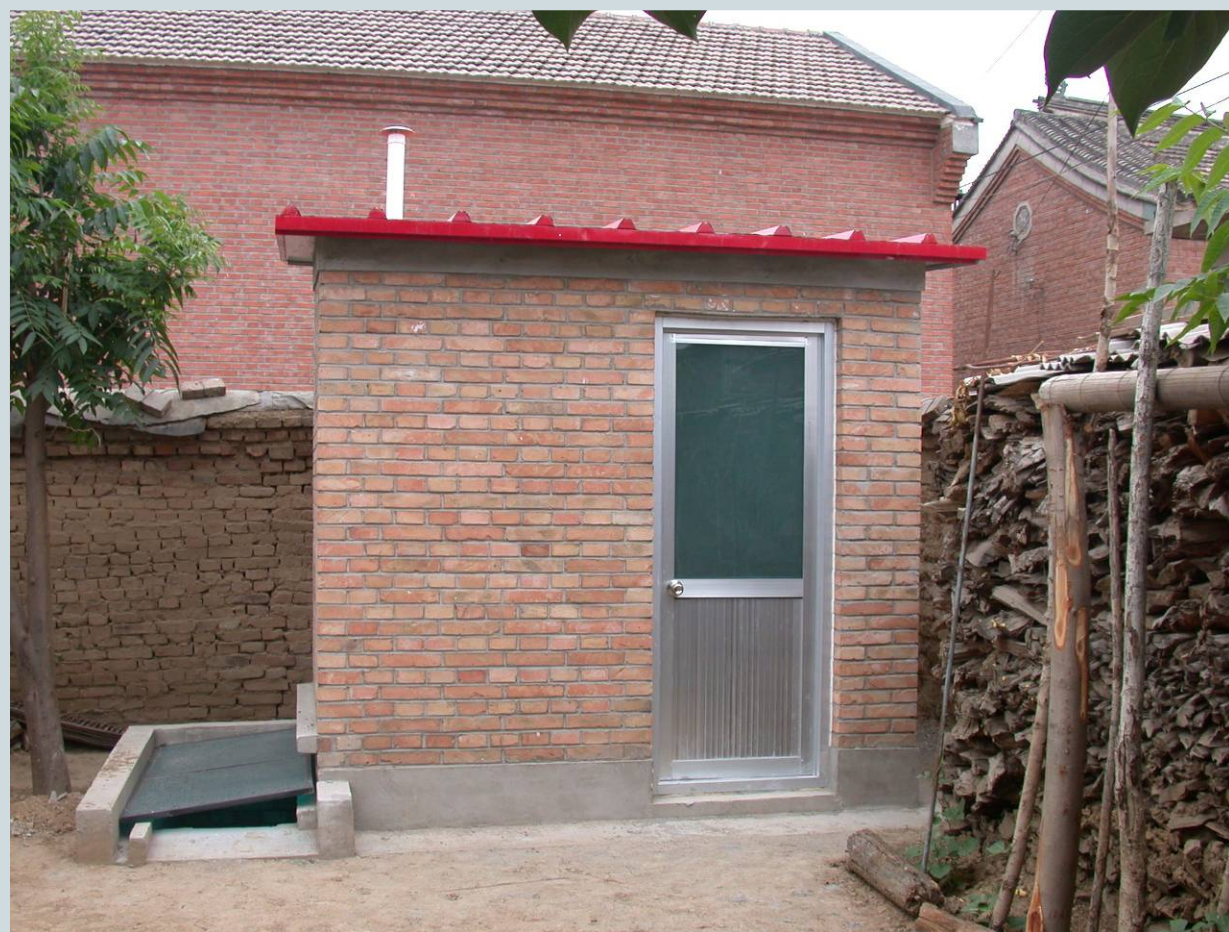
Before and after ecosan toilet renovation.
