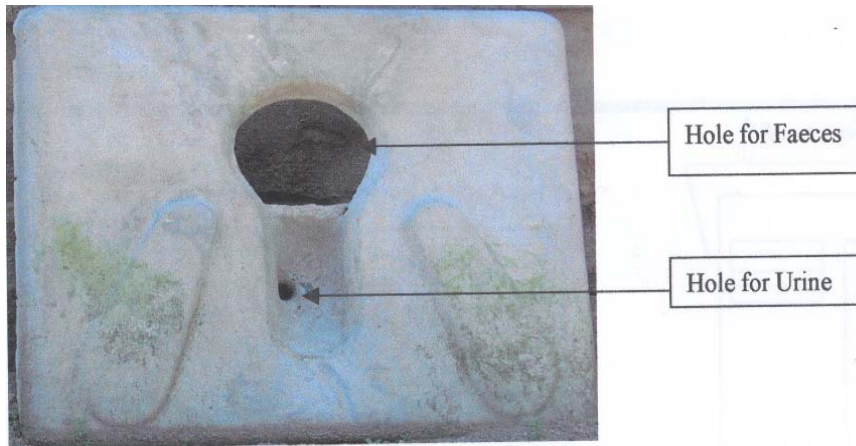
Picture 5: Detail B: Squatting-Pan
