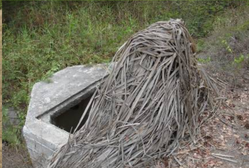
Abandoned Oxidation ponds
