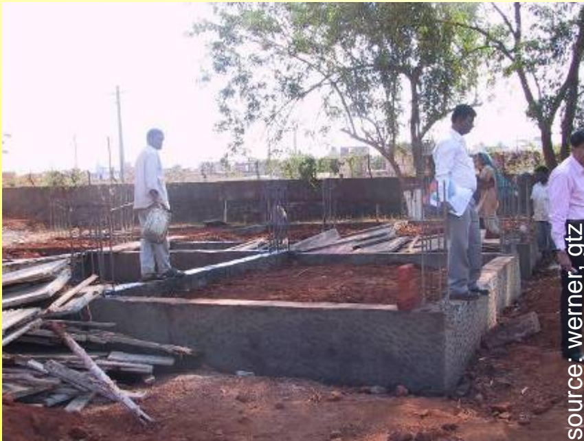
toilet center under construction
