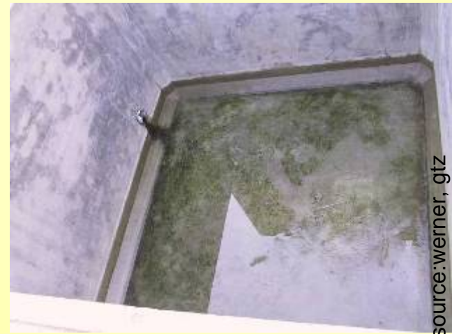
storage of treated greywater
