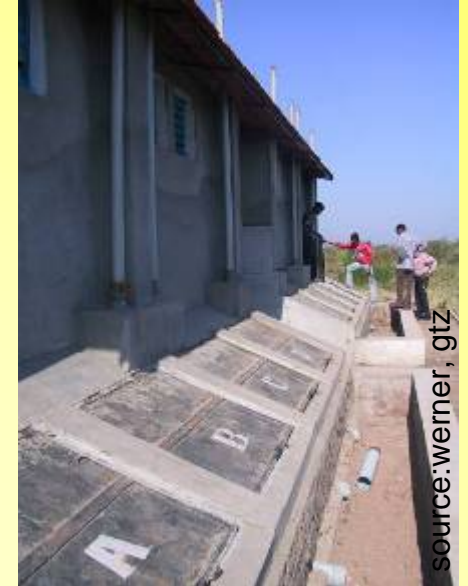
rear view of dehydration chambers
