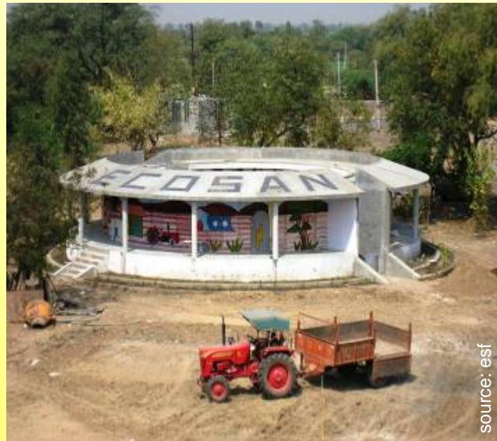
toilet block with biogas plant, almost finished, Feb. 2007
