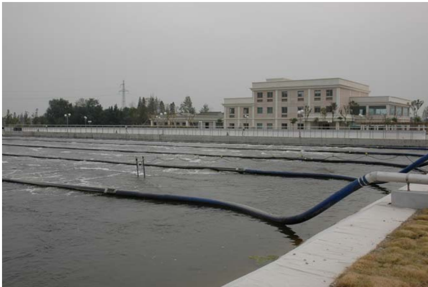
Gaoyou Sewage Treatment Plant
