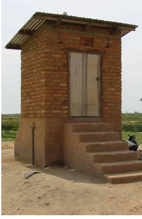
An Ecosan toilet in Ishasha
