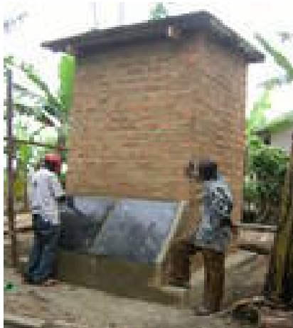
An Ecosan toilet in Ishasha
