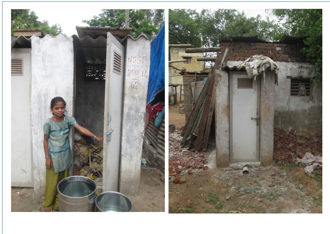
Figure 21: (Below Left) Unused IHHL; (Below Right) Inappropriate outlet for black water at an IHHL
