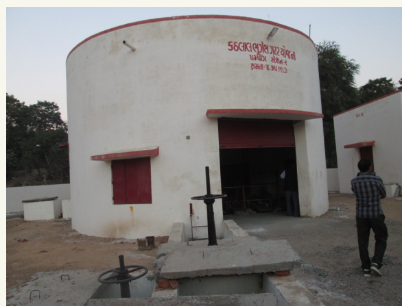
Figure 25: Pumping Station at STP in Kathlal, Gujarat
