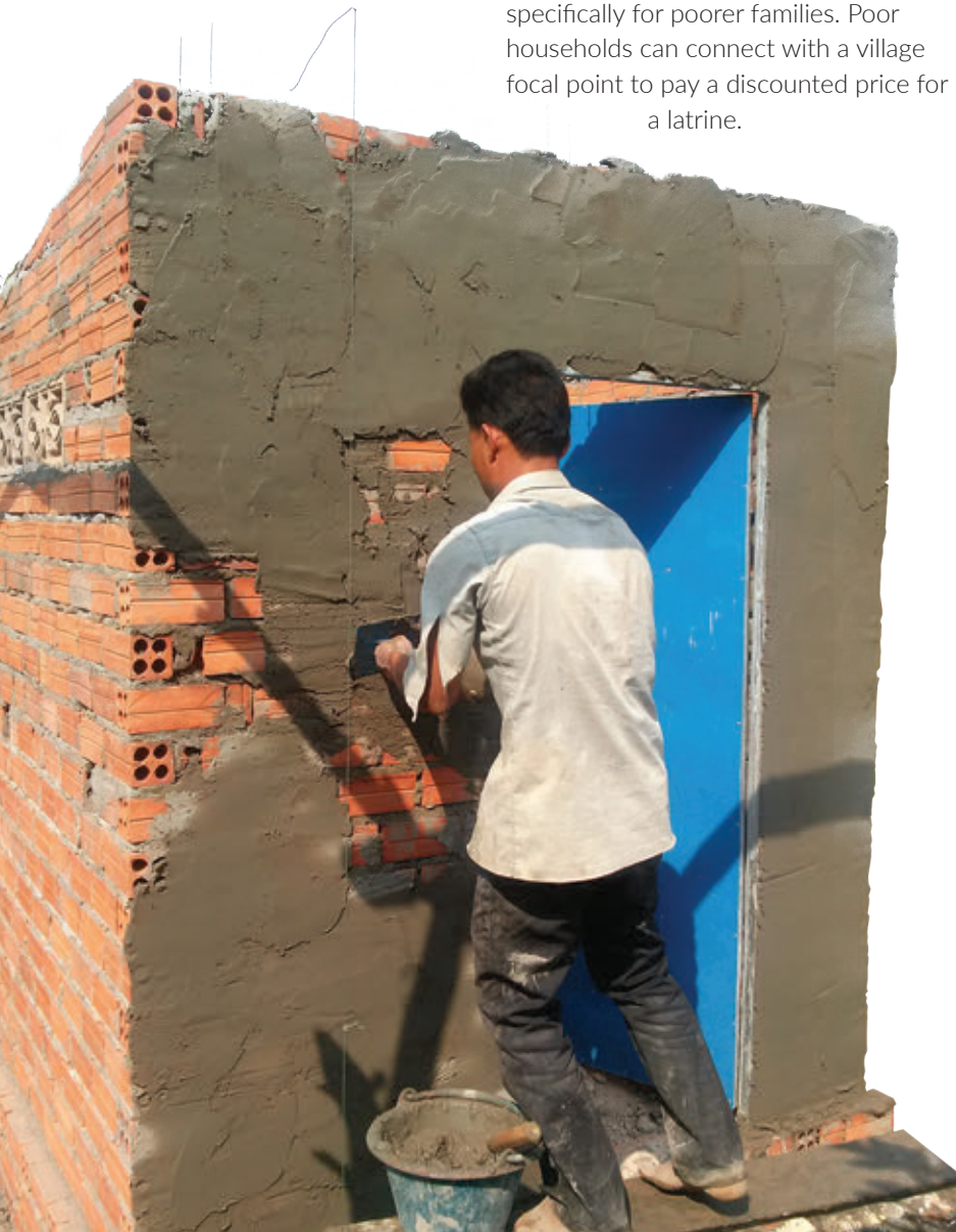
Local Mason working on the latrine construction
