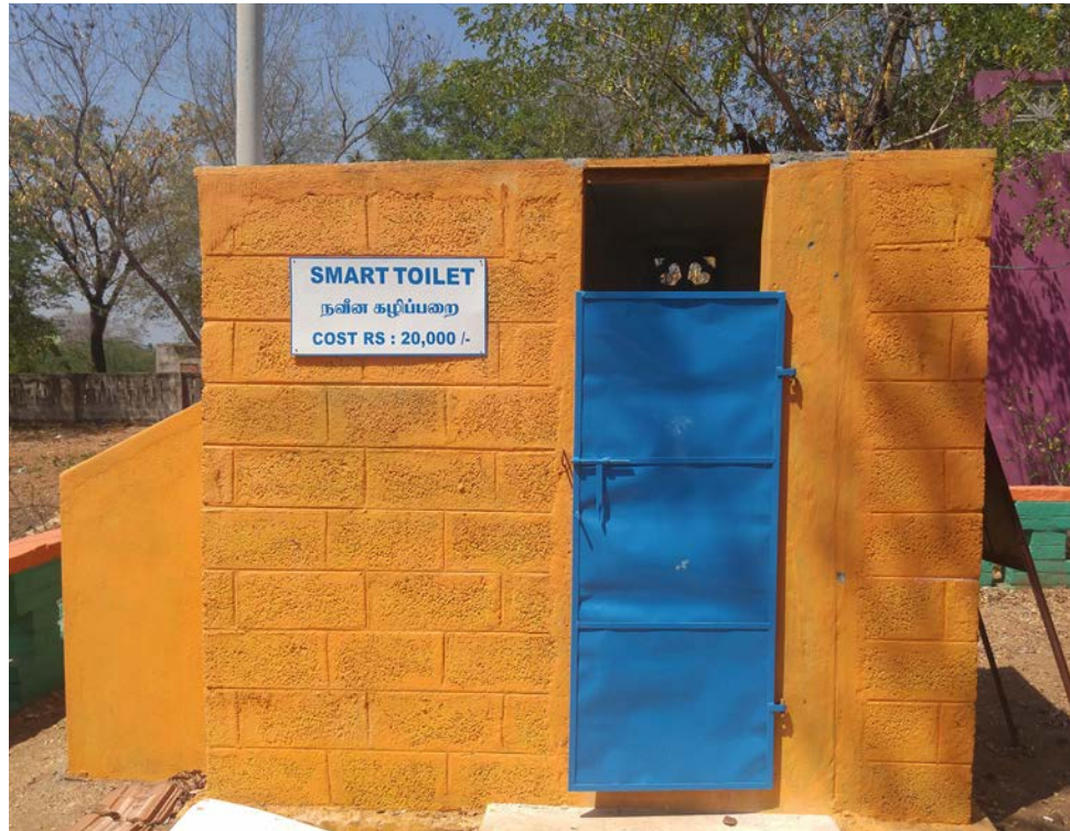
The SMART toilet incorporates twin pit latrines with a bathroom area to bathe in.
