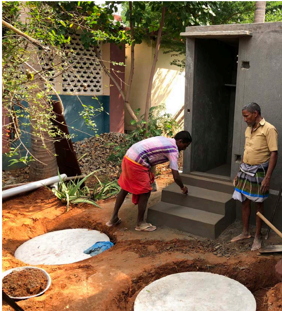
Masons building a twin pit toilet
