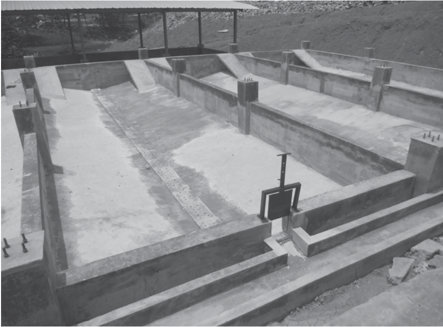
Photo 9.1 Drying beds under construction
