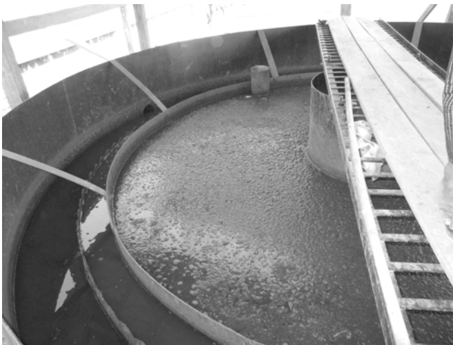
Photo 7.1 Hopper-bottomed gravity thickener, Sittwe, Myanmar Source: photo by Solidarités International
