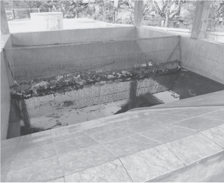
Photo 5.2 Vertical screen with no operator access
