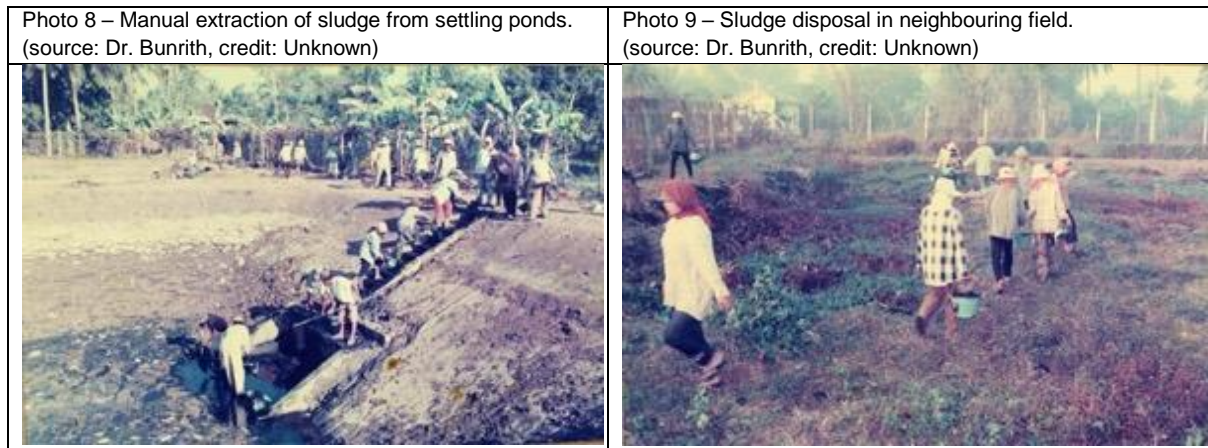
Figure 8: Photos of the cleaning of the Battambang WWTP sludge beds, circa 1995
