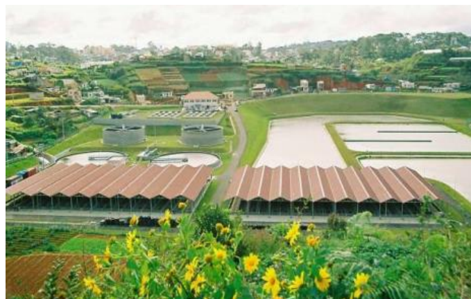
Figure 4: Wastewater Treatment Plant in Da Lat (Woo & Tran, 2013)
