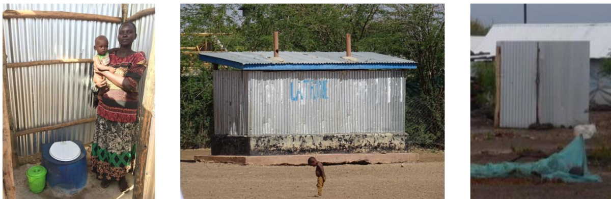
Figure 3: Toilets in Kakuma refugee camp (Sanivation hh toilet, communal toilet, NRC hh toilet)
