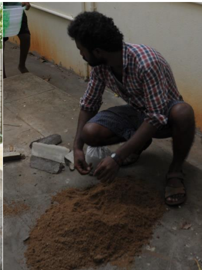
The lid of the tank is reconstructed by the workers.
