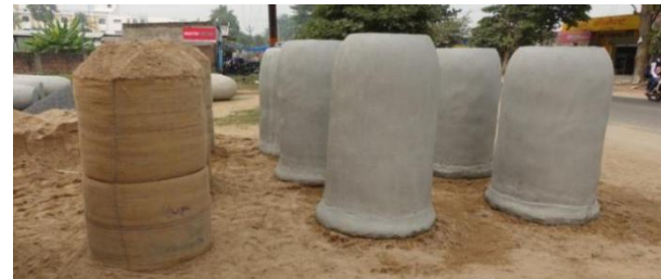
Figure 1: Prefabricated Septic tank (Source: Aishwarya /CSE, 2016)
