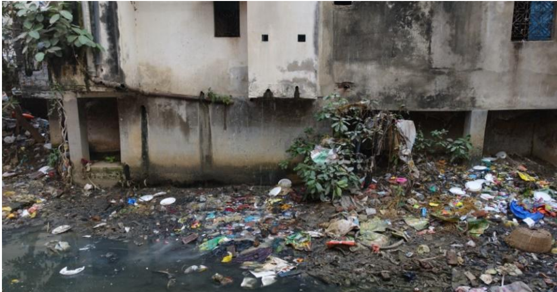
Figure 16: Direct release of sewage into Mocharim Pyne drain (Source: Aishwarya/CSE, 2016)
