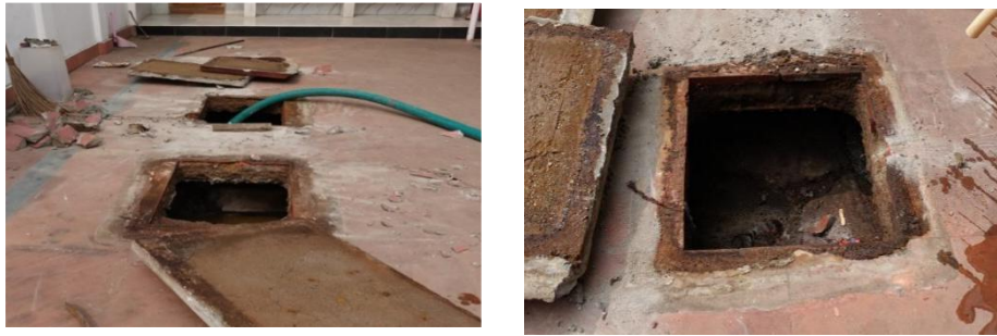
Figure 5: Emptying of a septic tank at the temple (Source: Shantanu/CSE, 2016)
