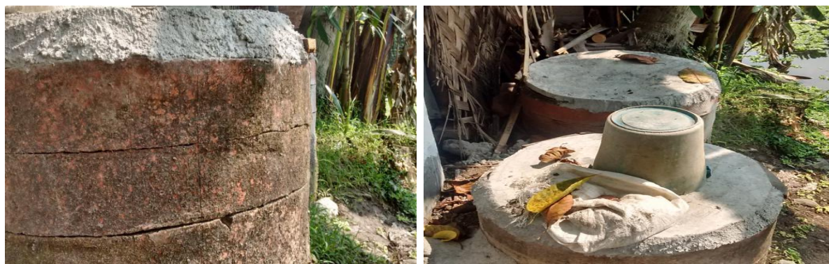
Figure 5: Twin-pit system (Source: Anil/CSE, 2016)
