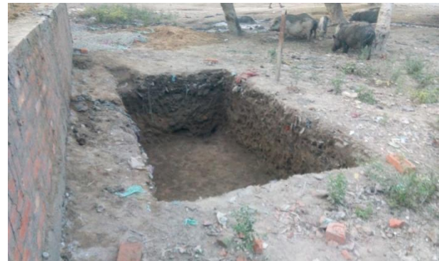
Figure 9: Septic tank of community toilet under construction at Ramrekha Ghat (Source: Amrita/CSE, 2016)
