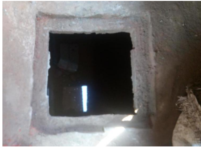
Figure 3: Newly constructed septic tank (Source: Amrita/CSE, 2016)
