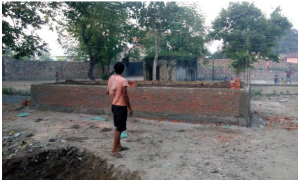
Figure 10: Under construction community toilet at Ramrekha Ghat (Source: Amrita/CSE, 2016)
