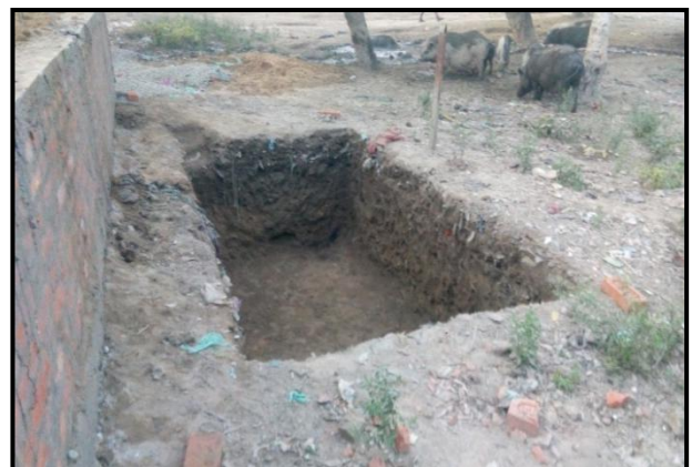
Figure 17: Containment system of community toilet at Ramrekha ghat in progress (Source: Amrita/CSE, 2016)
