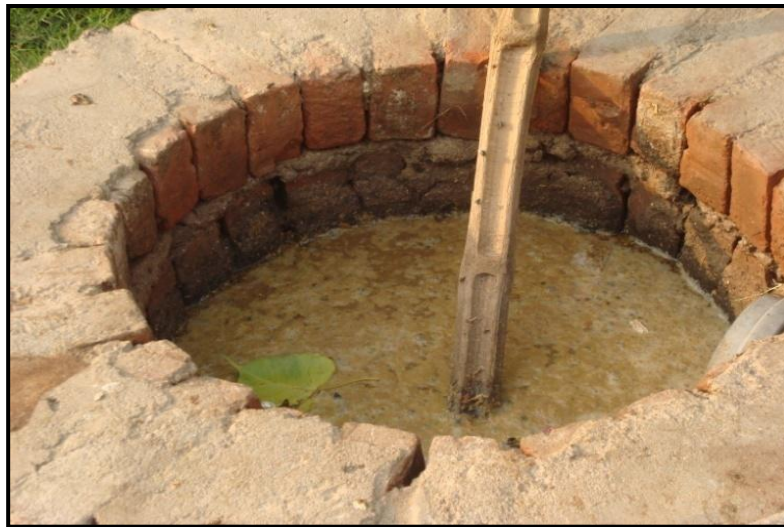
Figure 8: Pit used at the community toilet (Source: Amrita/CSE,2016)
