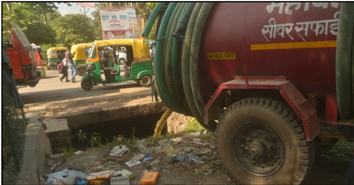
Figure 5: Emptying of sludge in open drains (Source: Anshul/CSE, 2016)
