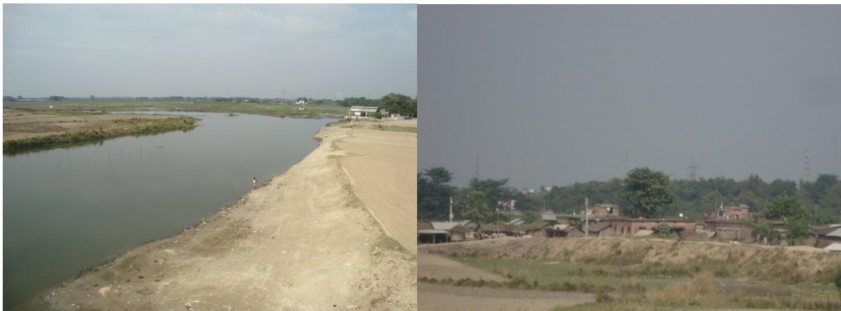
Figure 24: Kosi River and dam to prevent flooding (Source: Anil/CSE, 2016)
