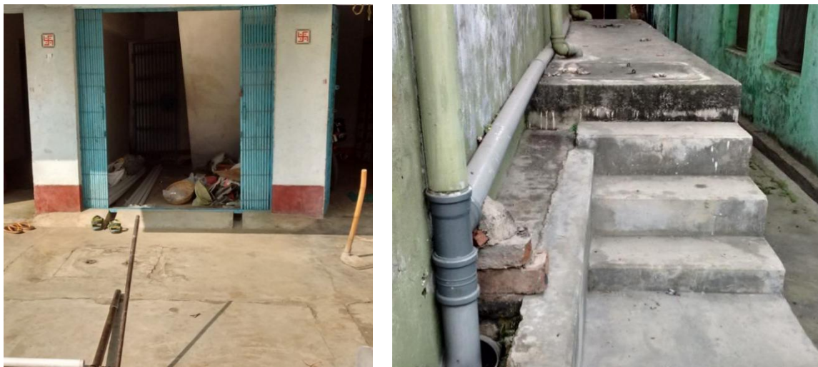
Figure 3: Septic tank in central area of the city (Source: Anshul/CSE, 2016)
