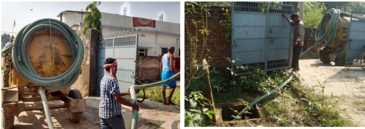
Figure 6: Emptying of soak pit containing SN from ST and grey water (Source: Anil/CSE, 2016)
