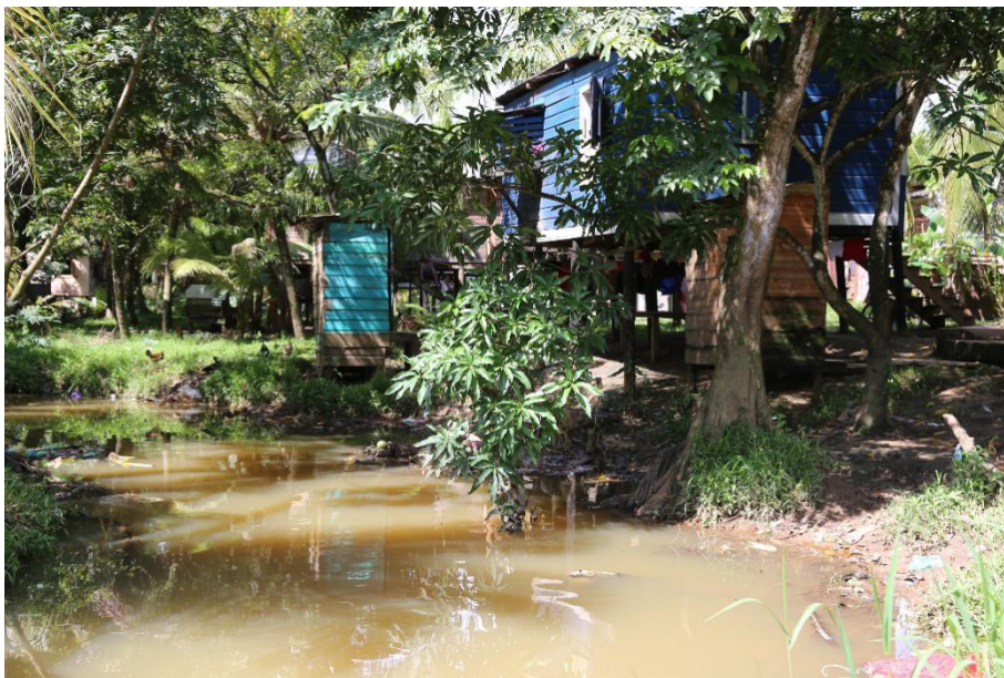
Figure 7: Hanging latrine over Bilwi Tingni creek (WaterAid/Eduardo Rodriguez 2018)
