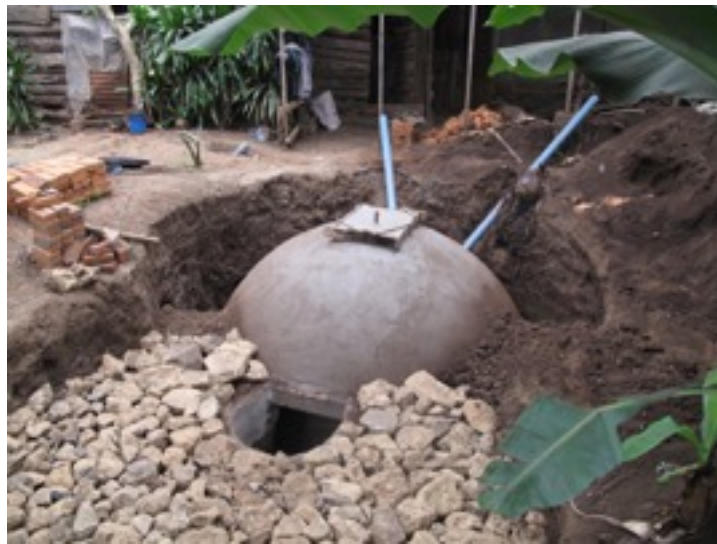
Figure 2.1: Bio-digester under construction: Arusha, Tanzania (Laramee, 2011) 6
