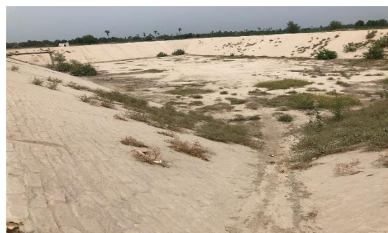
Figure 3: Treatment plant disposal point #2
