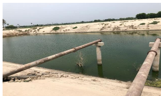
Figure 2: Treatment plant disposal point in Jatoi
