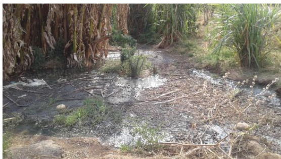
Figure 1: Sewage flow from burst pipe (Kamzati, 2018)
