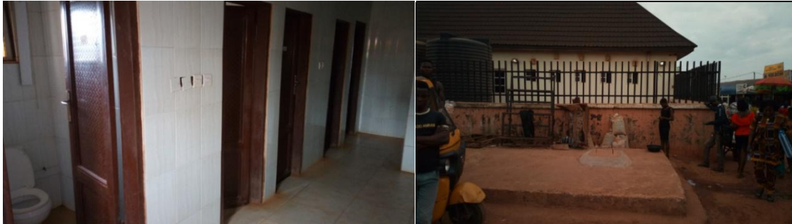
Figure 8: Inside and back view of the Ogbete Main Market Public Toilet (Photo credit: Chinedum Igwe)
