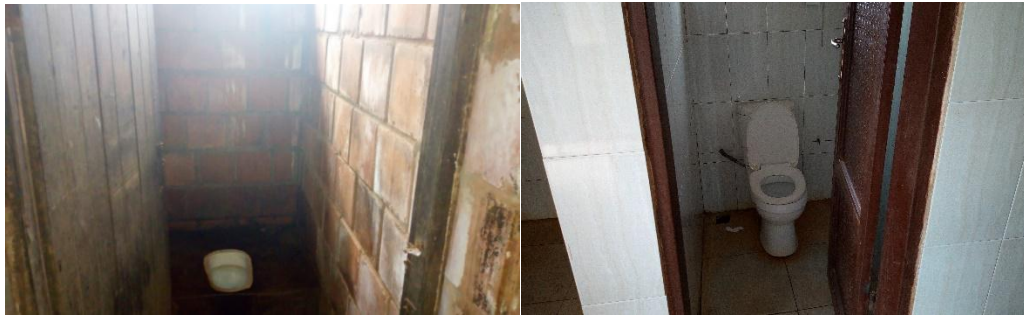
Figure. 3: A pour flush WC and an automatic flush WC (Photo credit: Chinedum Igwe)
