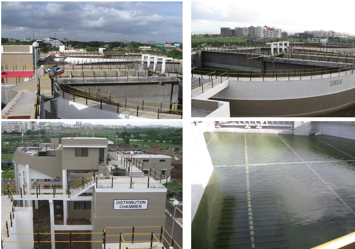
Figure 4 Kasarwadi- PCMC STP Plant
