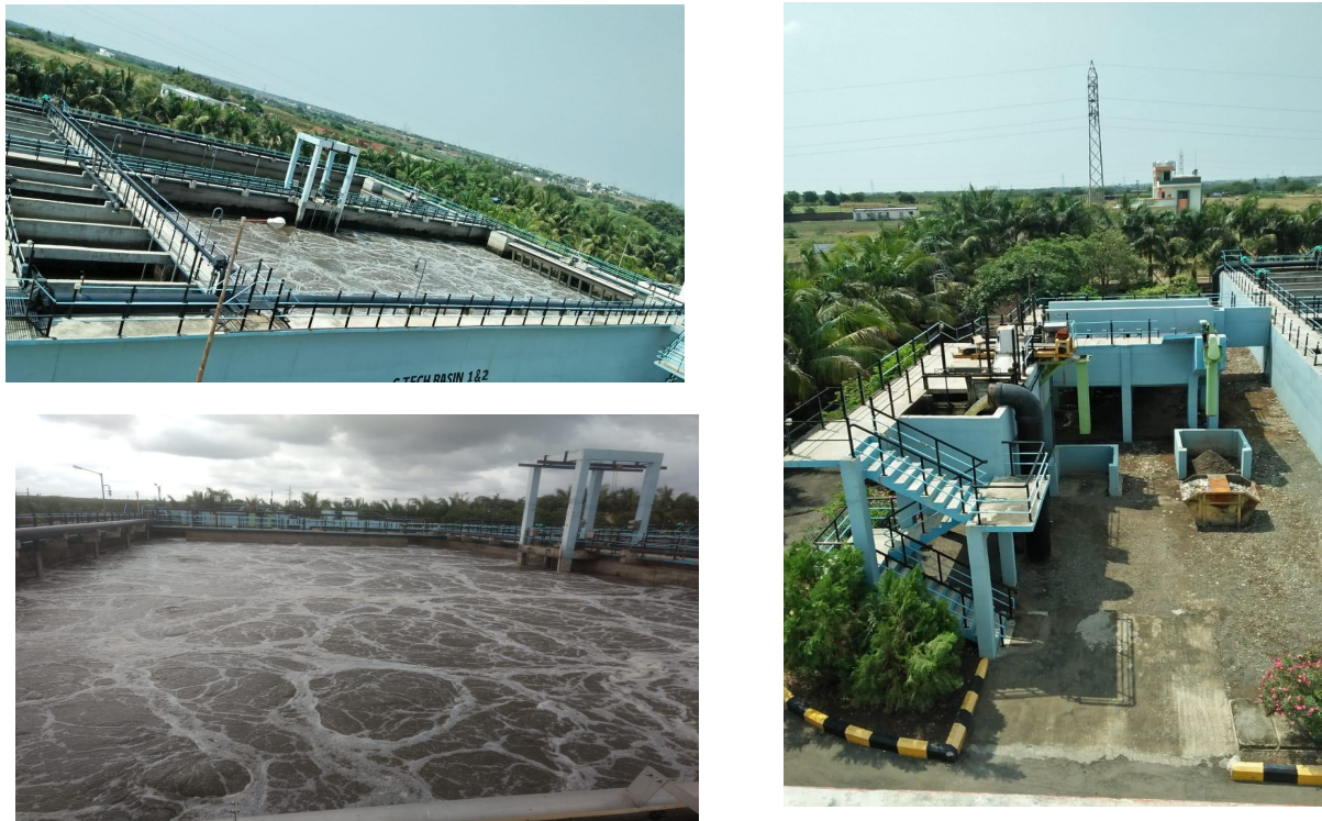
Figure 3: Pandharpur STP Plant
