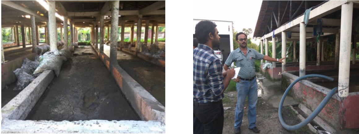
Figure 14: Sludge drying beds (Source: Aishwarya/CSE, 2016)
