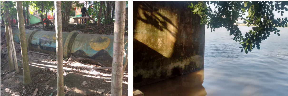
Figure 8: WW conveyed through big drain (Source: Aishwarya /CSE, 2016)
