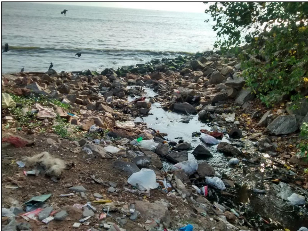
Figure 10: Storm water drains terminating in the Arabian Sea (Source: Bhavik/CSE, 2016)
