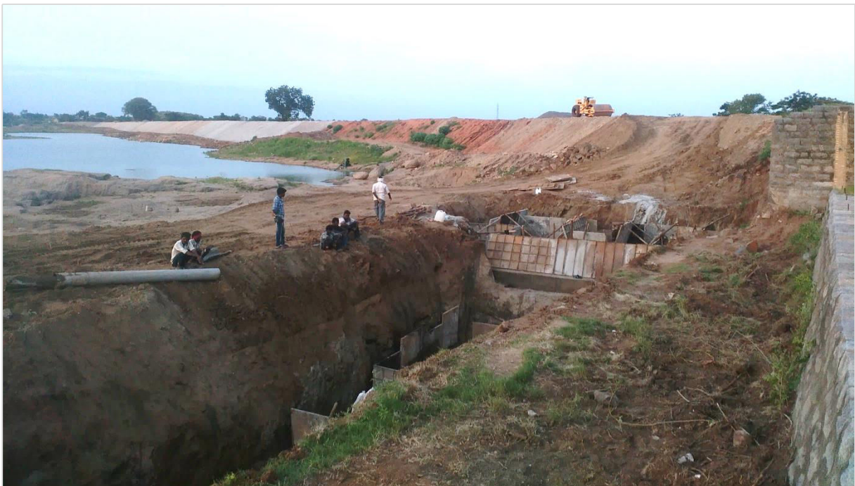
Figure 13: Proposed 24 MLD STP under construction (Source: Anil/CSE, 2016)
