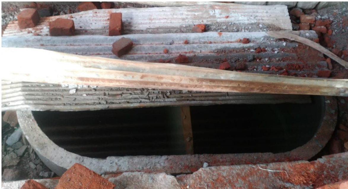
Figure 3: Septic tank under construction (Source: Shantanu/CSE, 2016)
