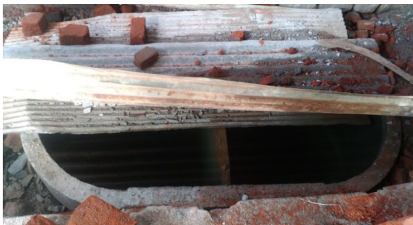
Figure 1: Cylindrical shape containment system (Source: Shantanu/CSE, 2016)
