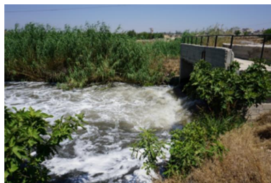
Picture 2: Outflow of waste water treatment plant
