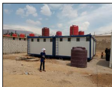
Picture 1: Typical school toilet installed for internally displaced persons
