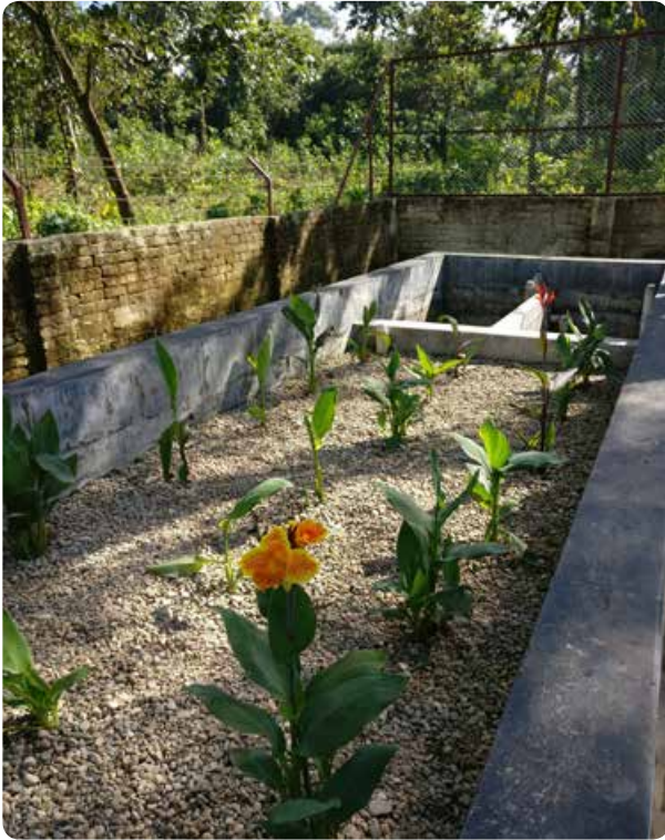
A constructed wetland and sludge drying beds in Sakhipur co-compost plant, Tangail, Bangladesh
